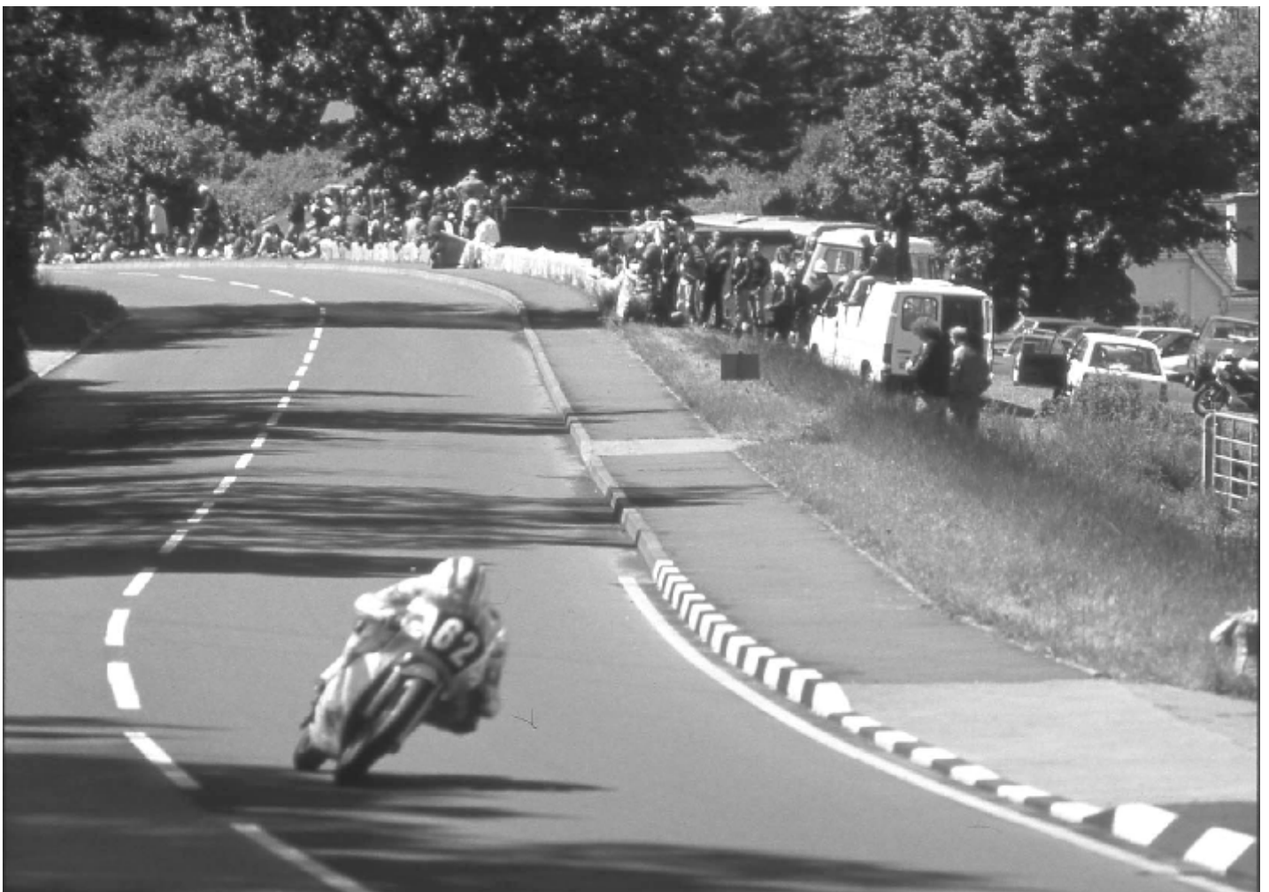
Re-surfaced Quarry Bends 1991,
